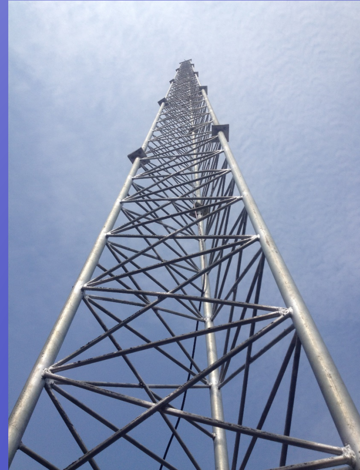
Sollinganallur Taluk VHF site, Kanchivaram, TN
